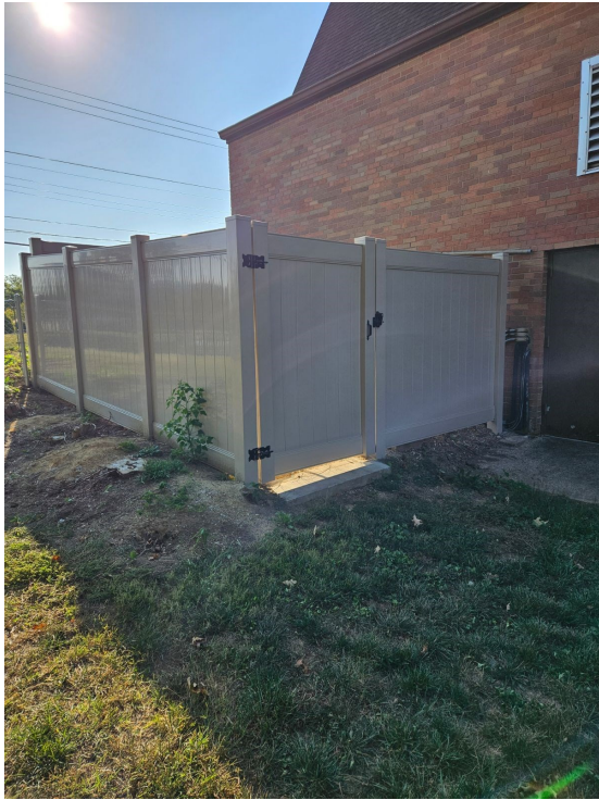
NEW PRIVACY FENCE FOR AIR CONDITIONERS
